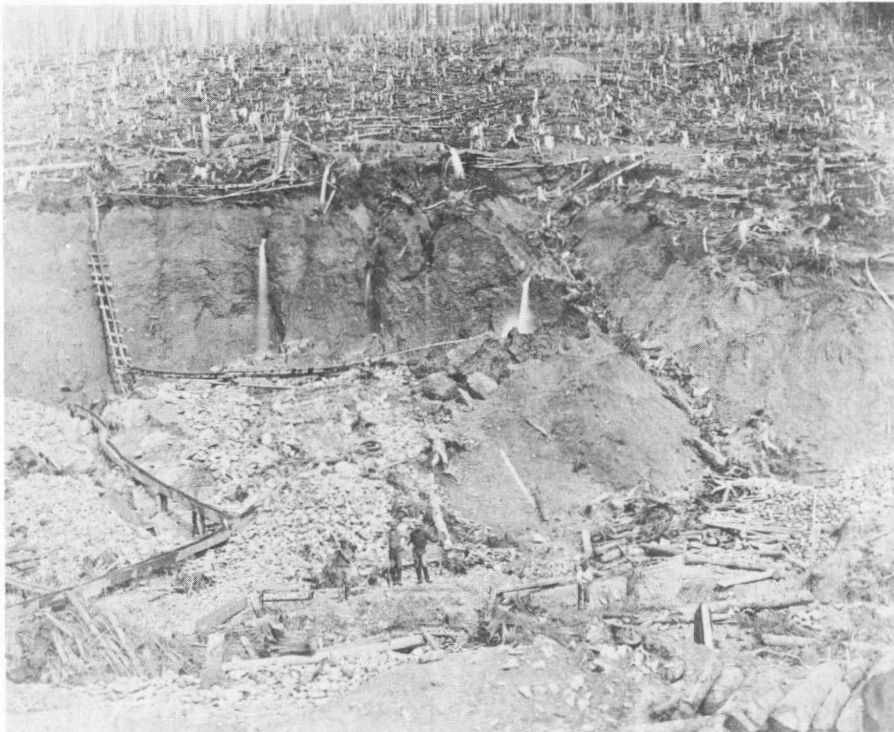
Hydraulic Gold Mining, Williams Creek, 1867-68. Frederick Dally. Panoramas taken at the gold fields reveal the havoc of truncated hillsides where miners posed proudly among felled trees, rock tailings, planks, barrels, ladders and sluice-boxes on their claims. (Public Archives of Canada C-26181)
