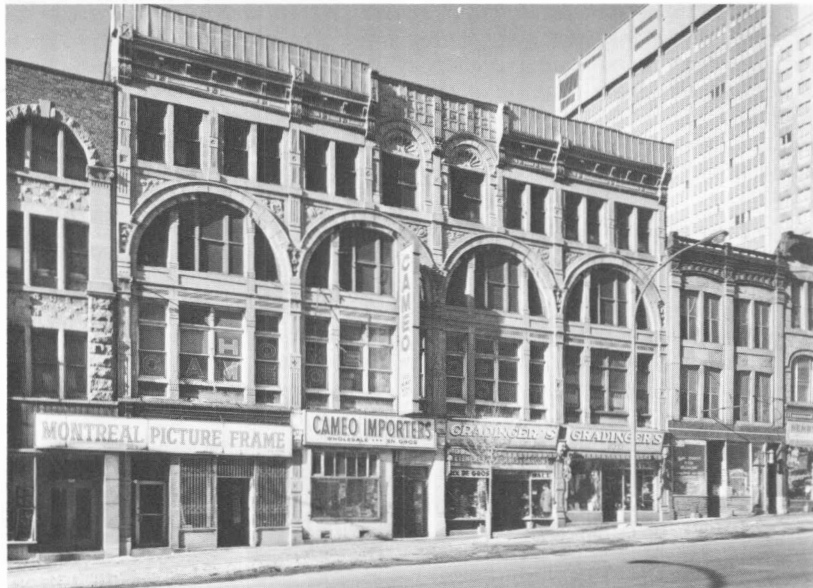
D.J. Ouimet Grocery Store and Dwelling, 1887: architect not known (901 rue Cherrier).
