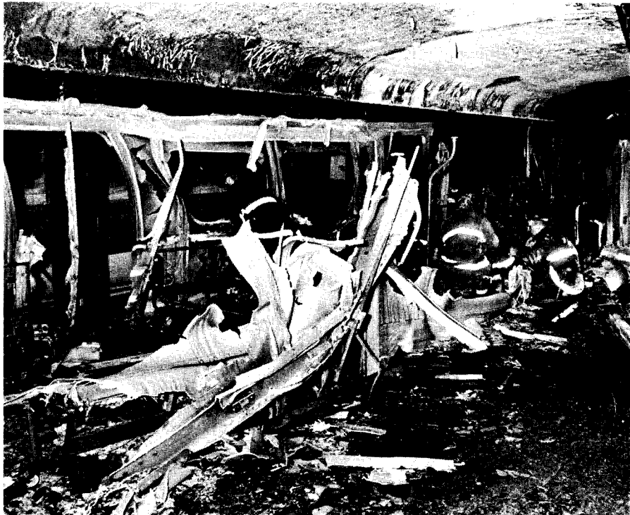
Melted subway cars after the 1976 Toronto Transit Commission subway fire. (Toronto Fire Department)
