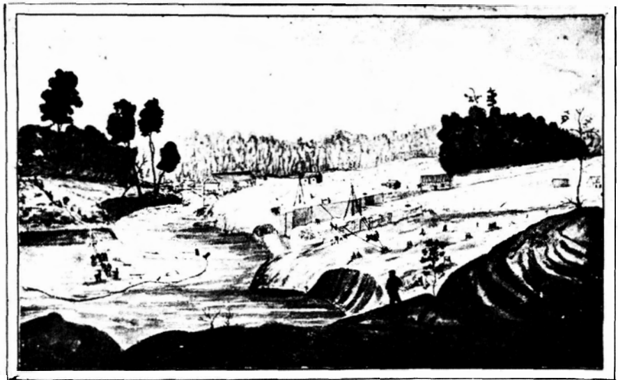
Figure 7: Thomas Burrowes, "Brewer's Lower Mill. Masonry of the Lock nearly complete. Excavation for Canal in progress 1831-2." Courtesy: Picture Division, Public Archives of Canada, C-11173.
