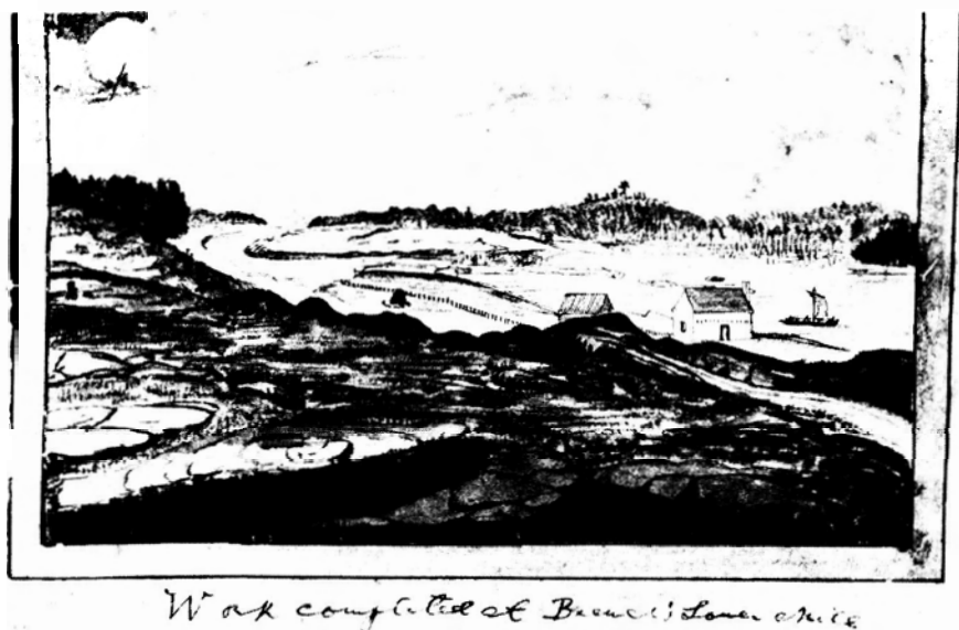
Figure 8: Thomas Burrowes, "Work completed at Brewer's Lower Mill," 1832. Courtesy: Picture Division, Public Archives of Canada, C-11174.
