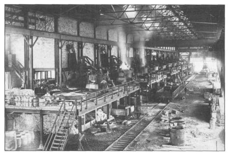
Figure 1: Interior of British Forging's melting house, showing two of the ten electric furnaces in operation on 28 June 1917 only days after the first steel was poured. Courtesy: Toronto Harbour Commission Archives, Arthur Beales Collection, PC 1/1/2859.
