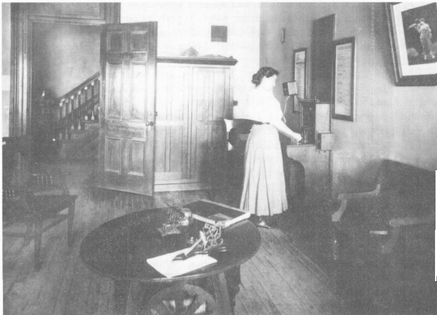
Figure 3: Switchboard, Asylum for the Insane, Brockville, Ont., c. 1906. Courtesy: Archives of Ontario, R.G.10 20-H.
