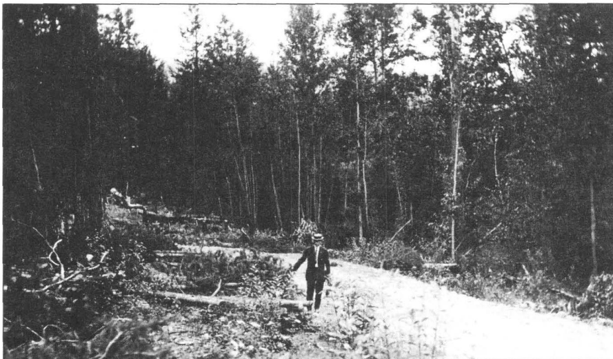
Figure 5 "Fire hazard along provincial government wagon road in southern British Columbia, due to failure of construction gang to pile and burn debris when building road. This condition is now being gradually corrected." (PA187139)
