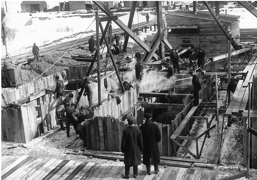
Figure 2 B.V. 417 Feb. 8, 1915 Progress Pier D (City of Toronto Archives, RG 8-10-417)
